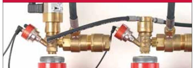
DIMES replaces passive pressure gauges for more accurate and pro-active monitoring as well as secondary functionalities.
